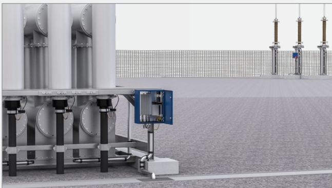
TE-Monitoring an Kabelendverschlüssen
