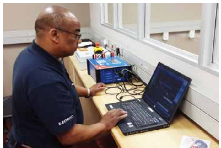
Keith Daniels, City of Cape Town, calibrating voltage and current transformers using VOTANO 100 and the CT Analyzer.
