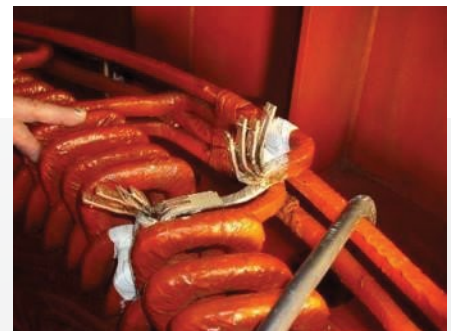
Repair of defective soldering contact
