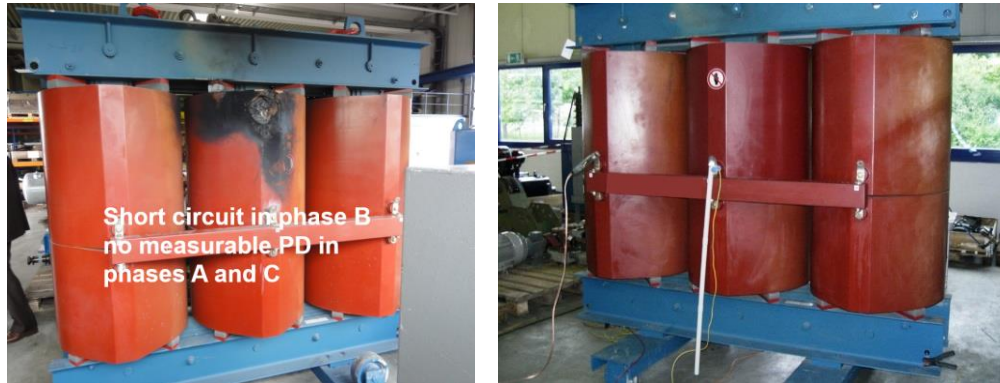
Fig. 16 2,5 MVA transformer before and after repair
